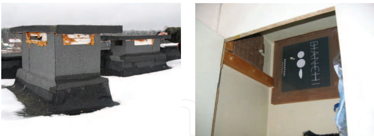
Fig. 4. Ventilation stack is closed by occupants due to cold air inflow caused by wind
