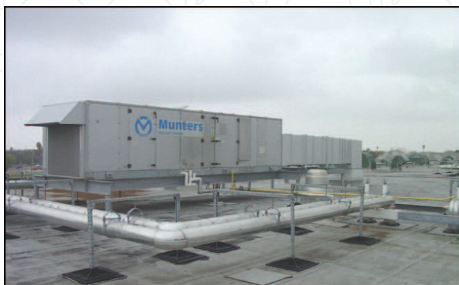
Fig. 1. Desiccant unit installed in a south Texas school to provide pre-conditioned fresh air for ventilation.
