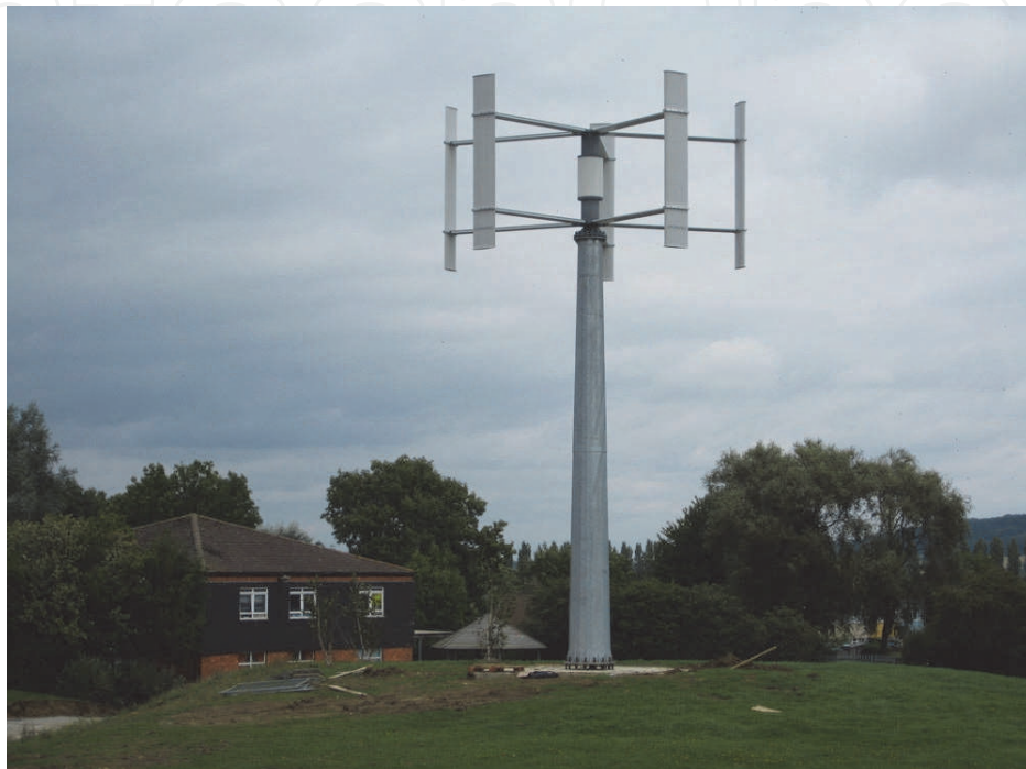
Fig. 4. H-type VAWT made by Ropatec of Italy
