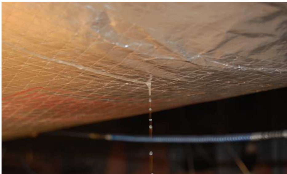
Fig. 10. Water running out of insulation.
