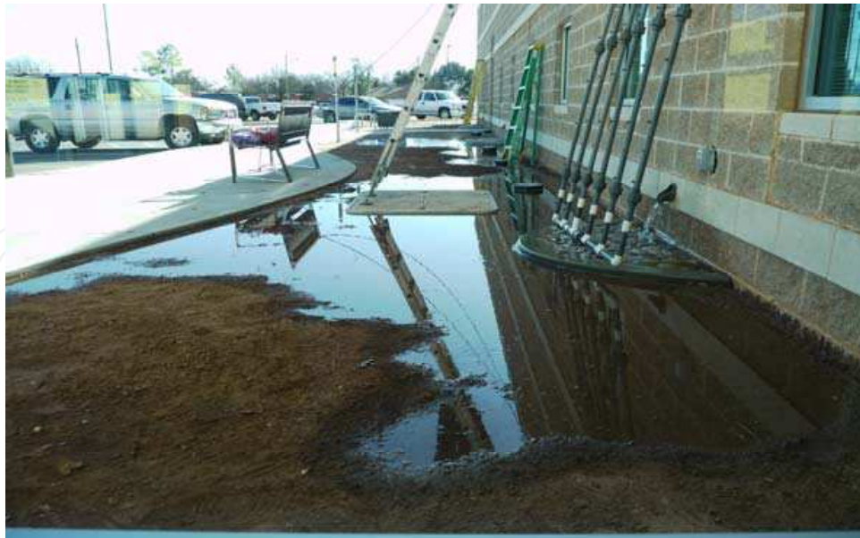
Fig. 11. Improper site grading.
