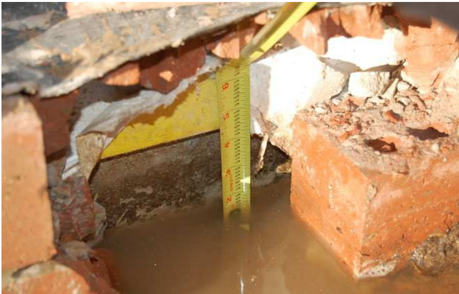
Fig. 9. Water standing inside the wall cavity.
