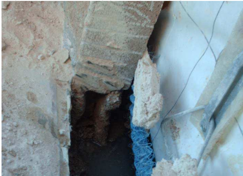
Fig. 12. Water standing inside wall cavity.
