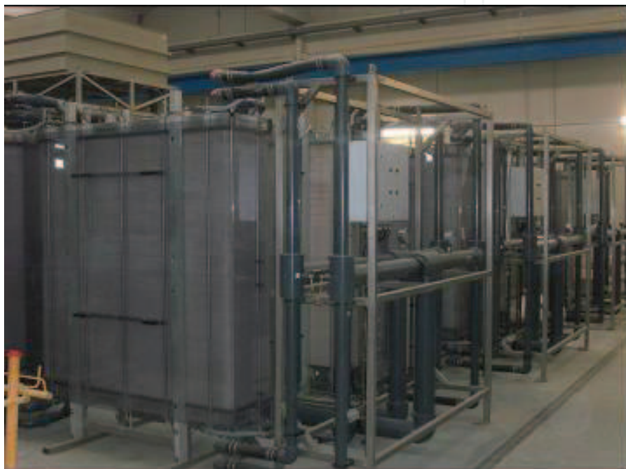
Fig. 4. EDR stacks at the Depurbaix WWTP.
