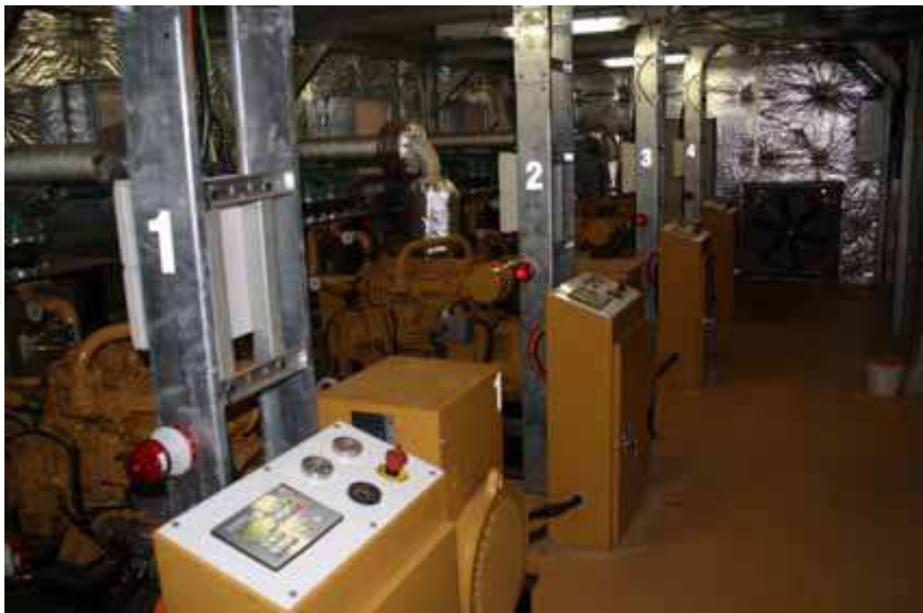
Fig. 19. Diesel Room at Eco Beach Resort
