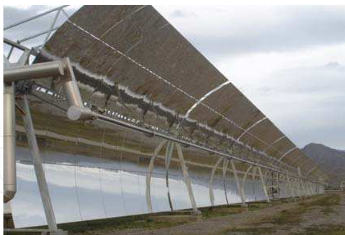
Fig. 3. Cylindrical parabolic concentrators at the PSA (Almería Solar Plant).
