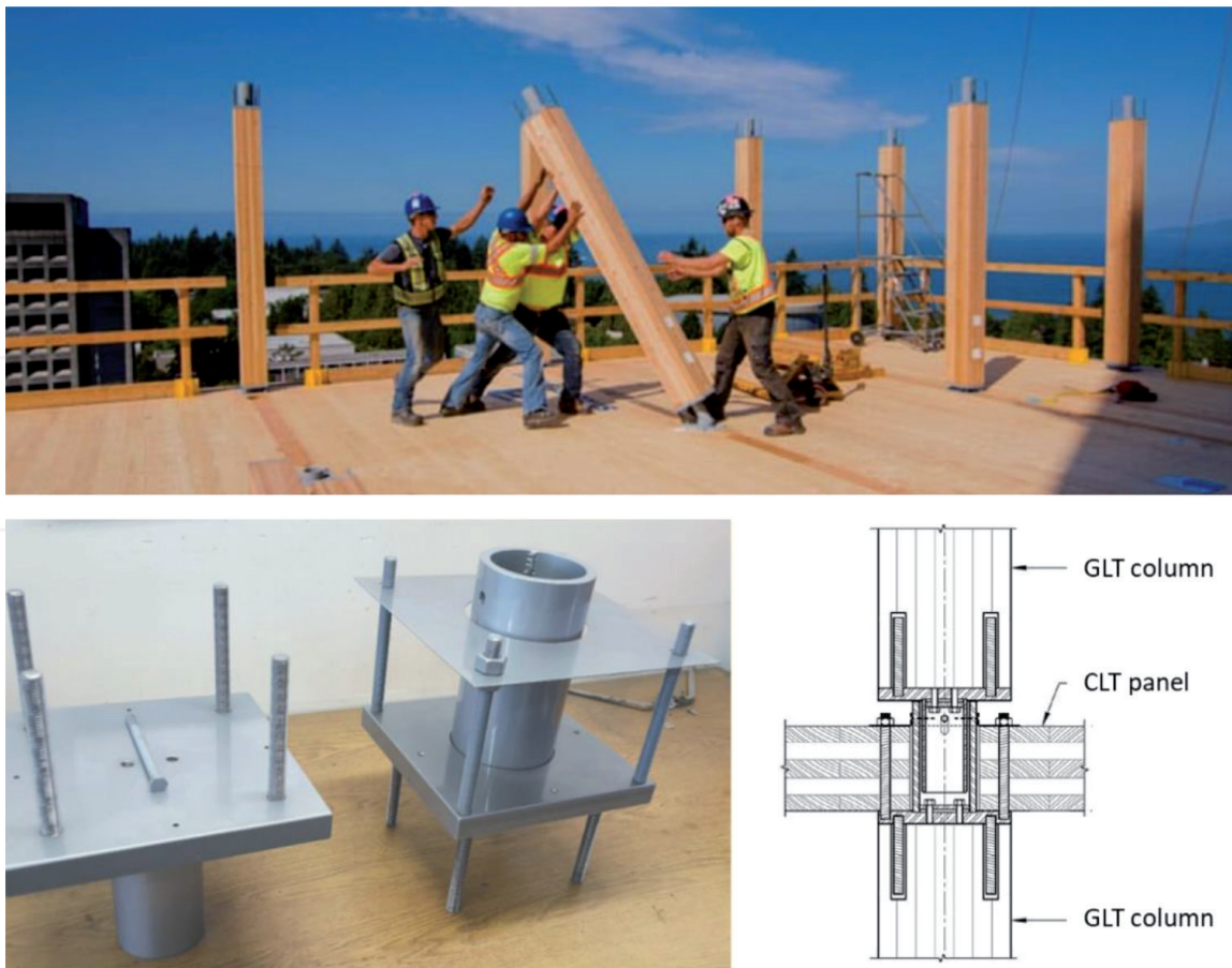
Figure 19. Column-to-column connection used in the Brock Commons Tallwood House in the University of British Columbia, Vancouver, Canada (upper: on-site installation of columns connected to CLT panels (source: www.fastepp.com ); lower: HSS steel connectors [26]).
