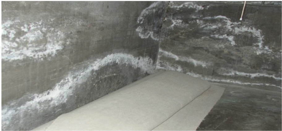
Figure 3. Excessive surface salt due to efflorescence phenomena.
