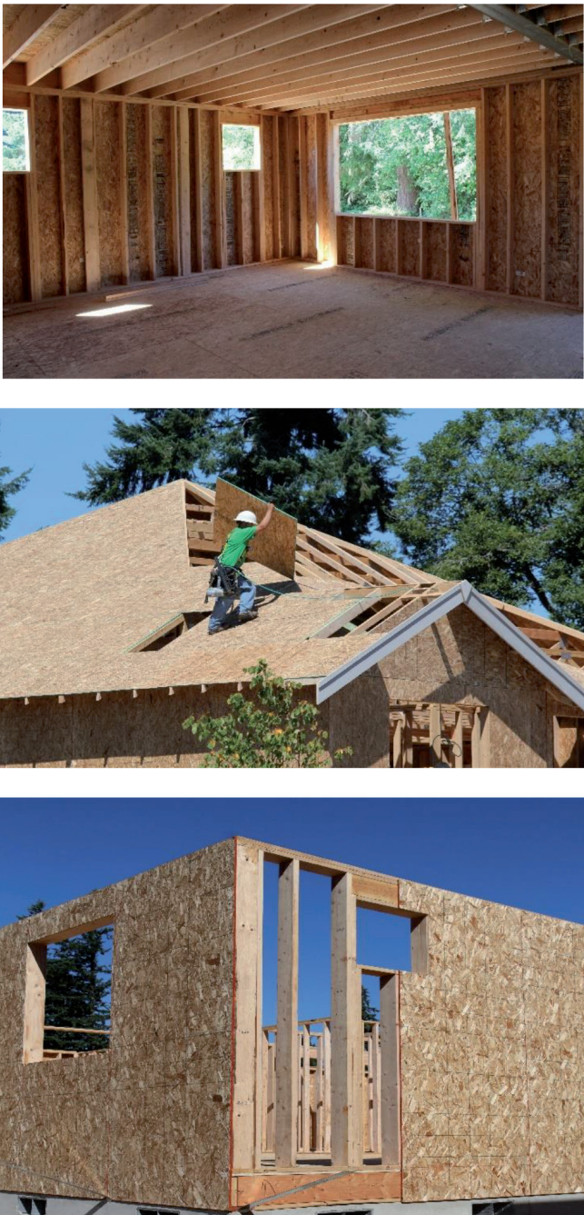
Figure 5. OSB sheathing used on floors (top), roofs (center), and walls (bottom) (source: Pictures obtained from APA at https://www.apawood.org/photography ).
