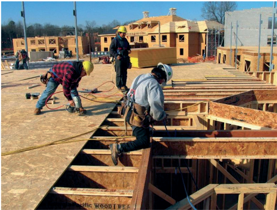
Figure 6. OSB used for floor sheathing and I-joist webs (source: Picture obtained from APA at https://www.apawood.org ).
