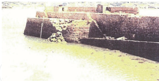
Figure 2. St Aubin's fort breakwater failure 1972 (archives).
