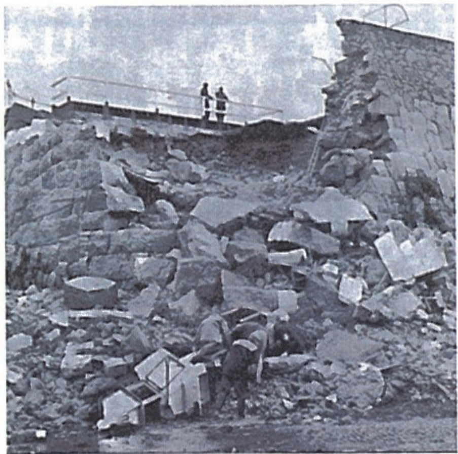
Figure 6. Collapse of Pierhead in 1965 (archives), Ref. [9].
