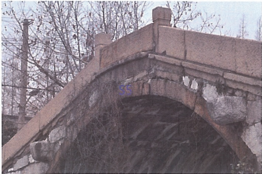
Figure 25. The damage to the slender Yongying bridge.
