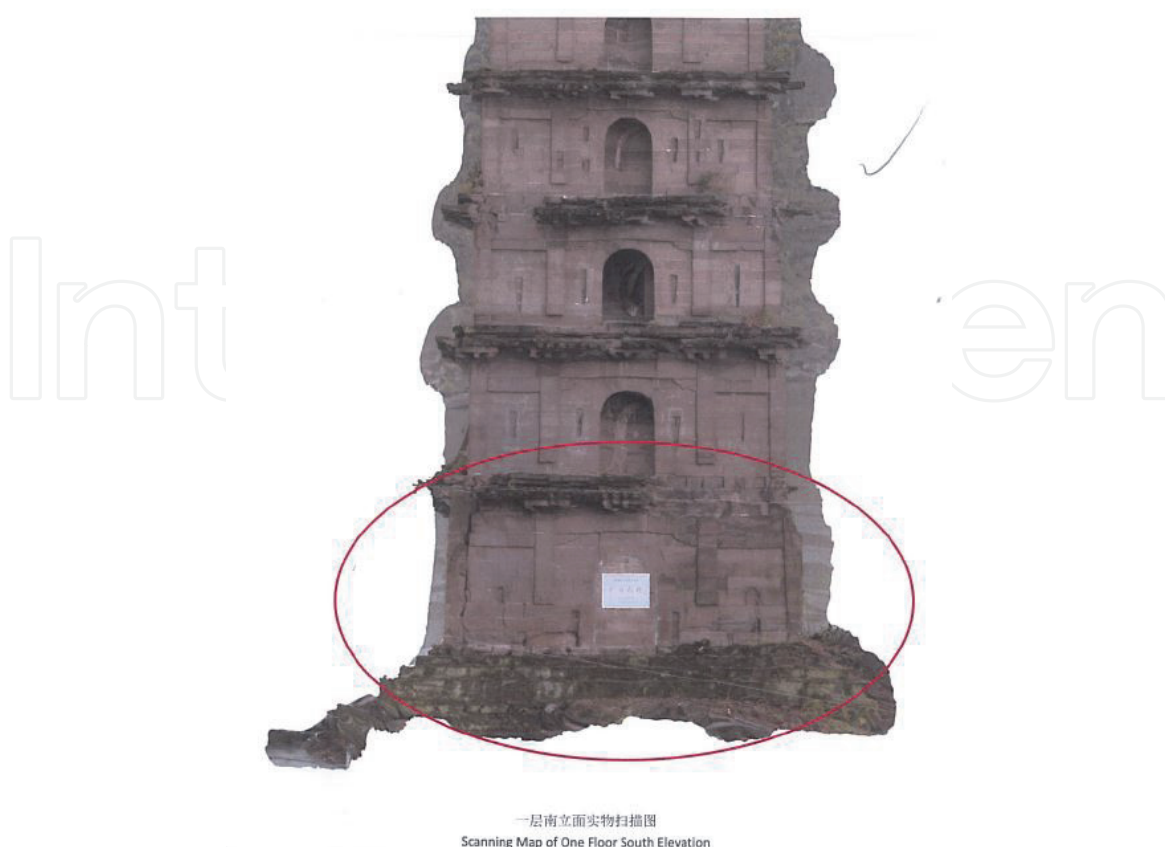
Figure 27. LiDAR scan of the white pagoda surface erosion.
