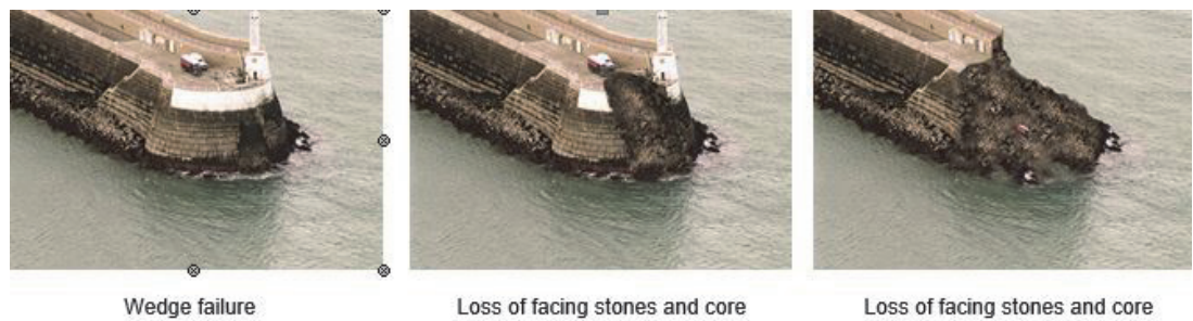
Figure 10. Photographic manipulation used to obtain emergency repair and protection funding, Ref. [11].
