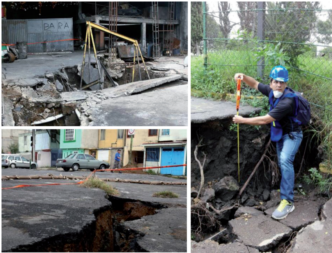
Figure 9. In the southeastern of Mexico City, where the poorest neighborhoods of the metropolis are concentrated, during the 2017 earthquake manifestations such as cracks, subsidence and collapses (steps) in the most superficial soils were exacerbated. This had the effect of the uninhabitability of thousands of homes. Since then, the city government undertook one of the largest reconstruction campaigns in the modern history of the city.
