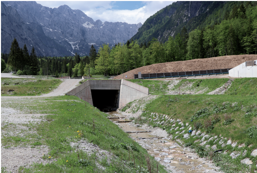
Figure 15. Regulation of the Nadiža torrent at the foot of the Planica ski-flying hill (photo: Jurij Beguš).
