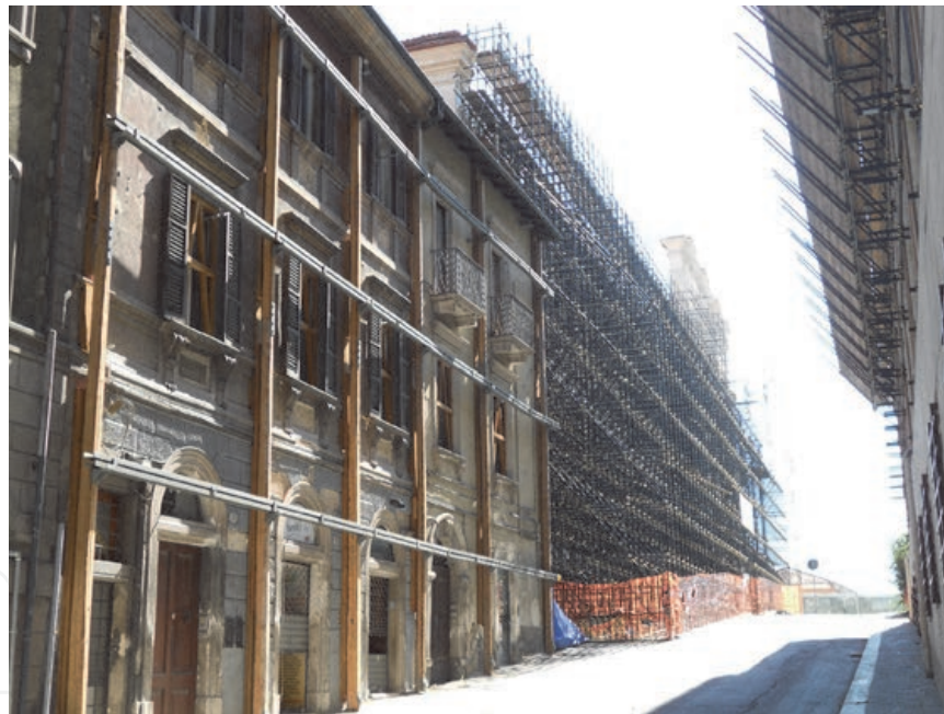
Figure 10. Props of different types along via di San Bernardino (photo S. Gizzi, 2011).
