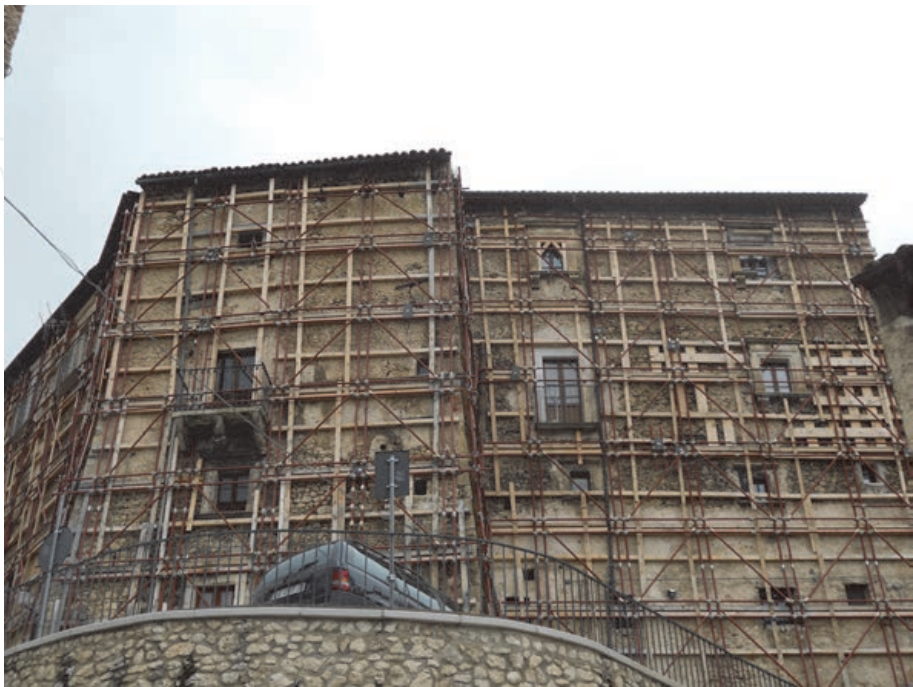
Figure 16. Provisional wooden work and props in the Medici center of Santo Stefano di Sessanio, near L'Aquila (Photo S. Gizzi, 2011).
