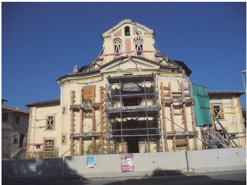
Figure 14. Emergency provisional works in wood in the church of Paganica (photo S. Gizzi, 2011).
