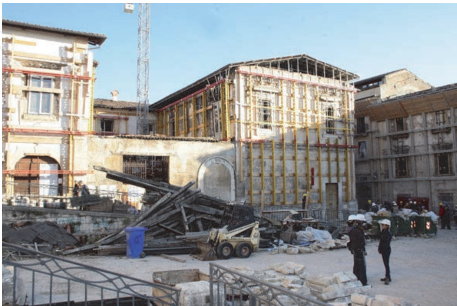
Figure 18. Props, temporary coverings and temporary works of various kinds in the square of San Pietro di Coppito in L'Aquila (photo S. Gizzi, 2010).
