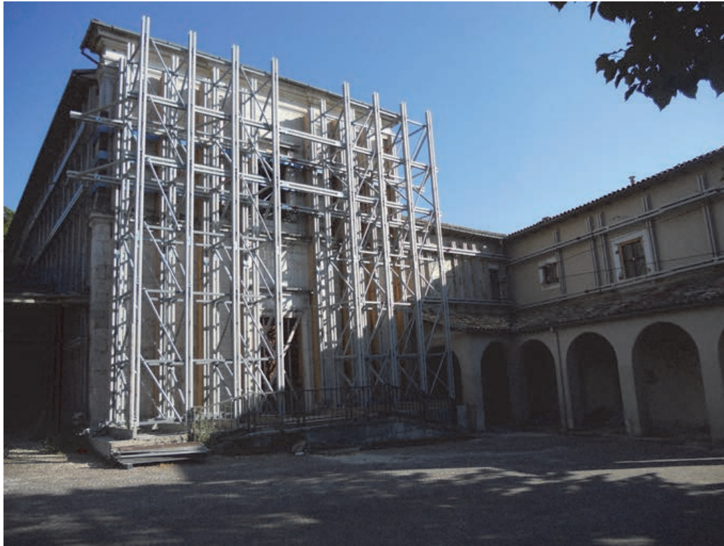
Figure 11. Shoring of the church of the Convent of Santa Chiara (photo S. Gizzi, 2011).
