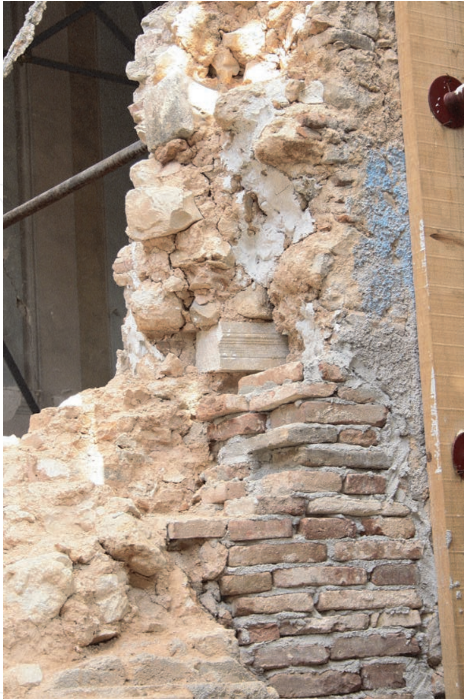
Figure 37. L'Aquila, church of Santa Maria Paganica. Reused stone elements that came to light inside the eighteenth-century walls after the collapse (photo S. Gizzi, 2010).
