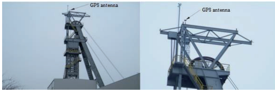
Figure 6. Head frame of S1.2 shaft, LW Bogdanka coaliery.
