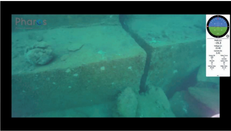
Figure 5. Quay blocks joint detail. Foundation footing.
