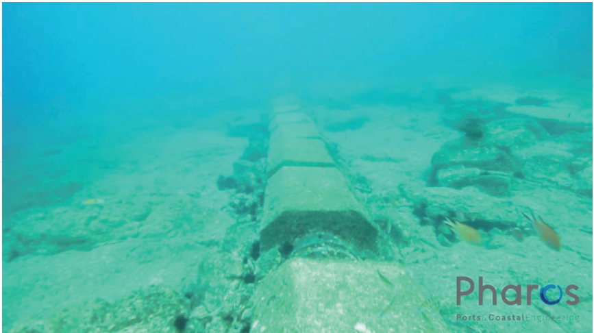
Figure 22. Detail of the concrete weights in a pipeline section near the coast.
