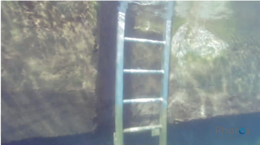
Figure 8. Lip finish of superstructure in submerged area.
