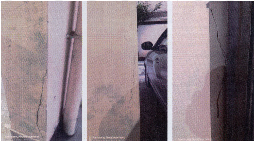
Figure 5. Typical distress in ground level columns caused by rust in ribbed TMT bars in a 10 year old building in Kolkata.
