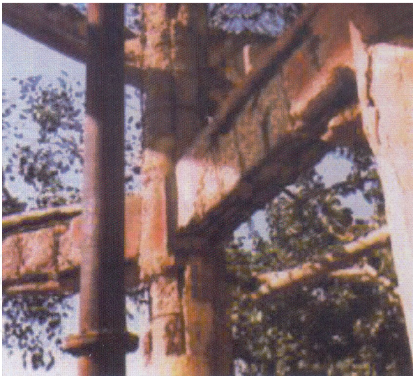
Figure 3. Distress in staging of overhead water reservoir due to corrosion in rebar.
