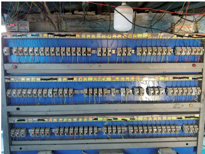
Figure 6. A miniature circuit breaker board of a neighbourhood diesel generator (Source: Author).
