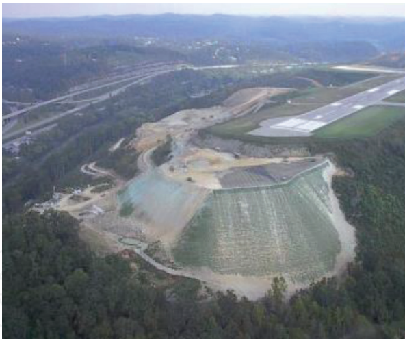
Figure 3. Reinforced slope Yeager runway extension (after [5]).
