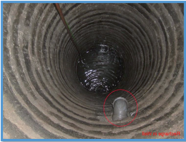
Figure 4. Dug well groundwater recharge structure.
