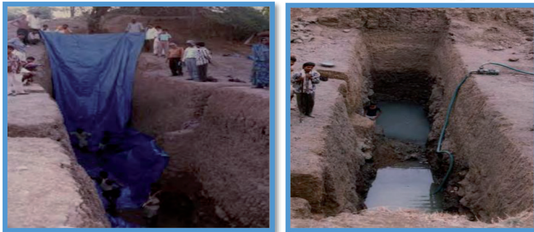
Figure 9. Artificial groundwater recharge structure at Rajgarh district in MP.
