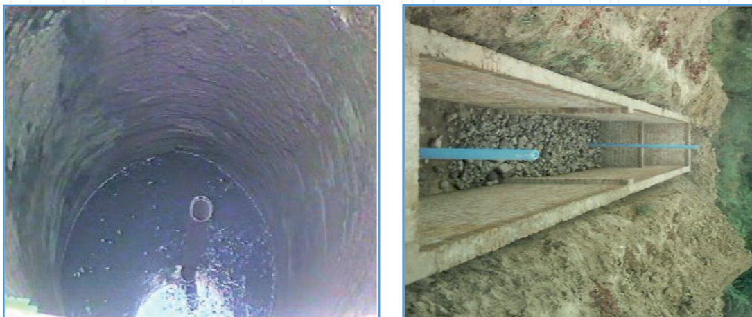
Figure 8. Artificial groundwater recharge structure at President's estate.
