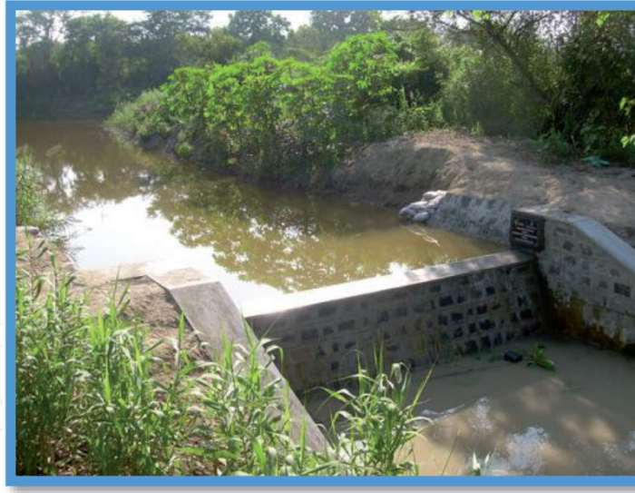
Figure 3. Check dam for surface water harvesting.
