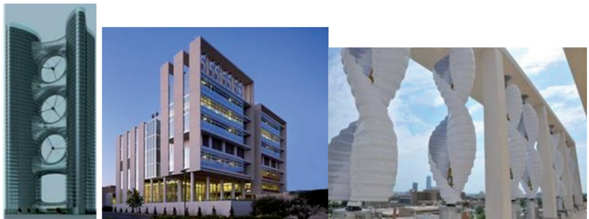
Figure 10. Wind turbines integrated into the building [20, 21].
