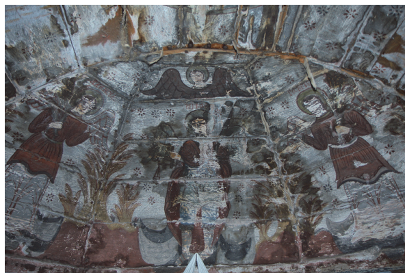
Figure 5. Semicap altar—degradation caused by humidity infiltration.
