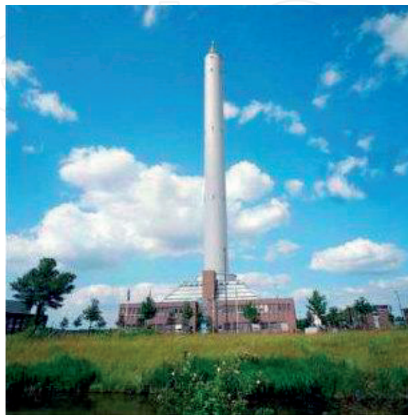
Figure 10. The ZARM drop tower in Bremen, Germany. The 146 m high building protects the free fall facility from atmospheric perturbation and wind (photo credit: ZARM).
