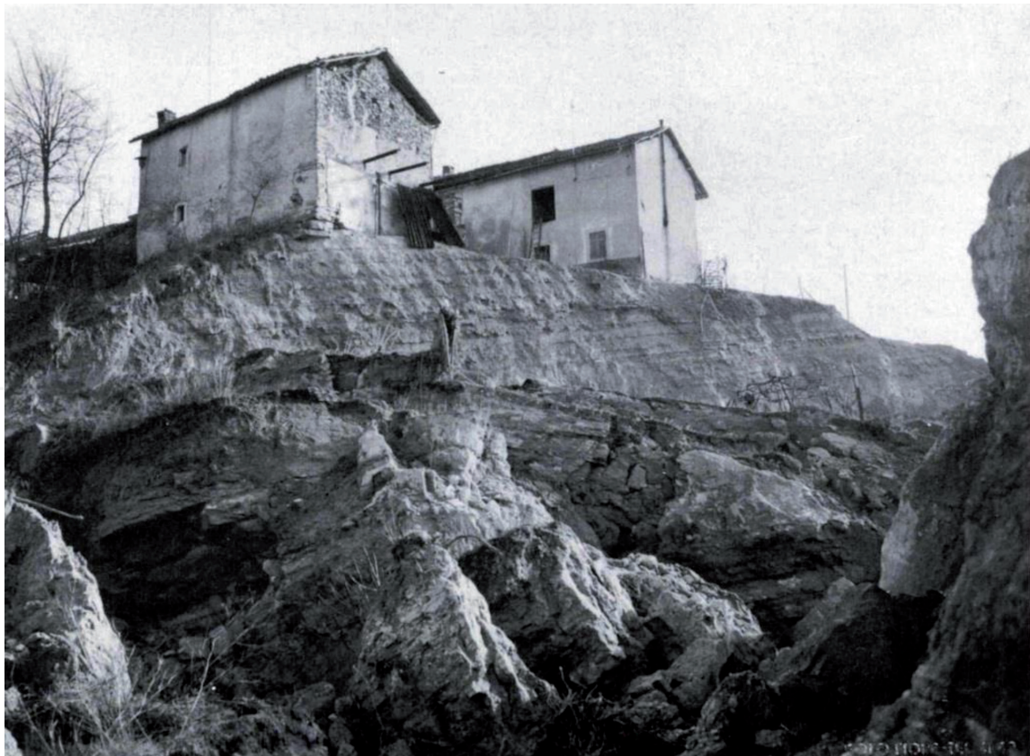
Figure 4. Detail of the landslide phenomenon of January 1963 in the crown area, in a photograph of the time. There are clearly visible bedrock structure dip slope of tertiary-age sedimentary rocks (on the left) and part of a slipped clod (on the right).
