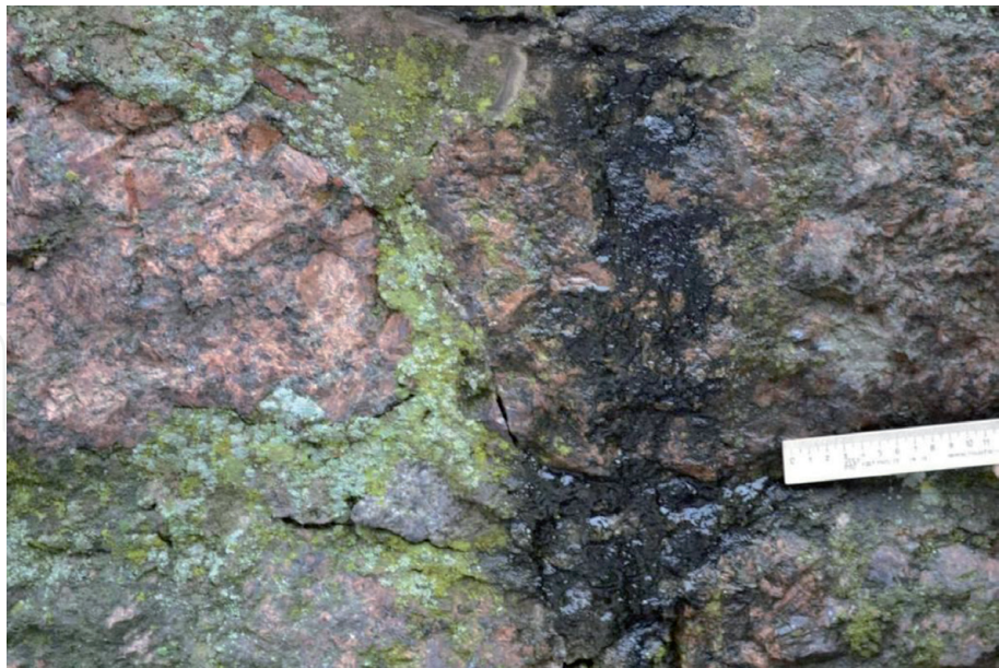
Figure 3. Biofilm formed by the cyanobacteria Microcoleus vaginatus Gomont ex Gomont on the granite wall of the Vyborg castle (Vyborg).
