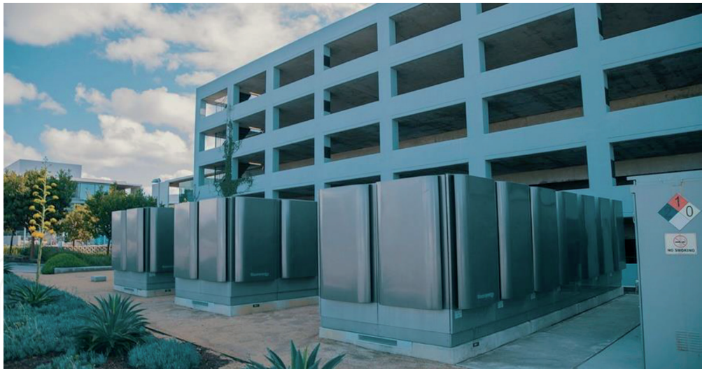
Figure 7. Fuel cells used at the La Jolla Commons building.
