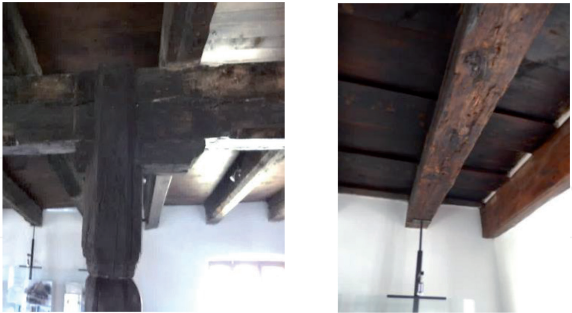
Figure 4. Supporting using a wooden beam and column (left) and ceiling wooden beam with a wooden decking (right).
