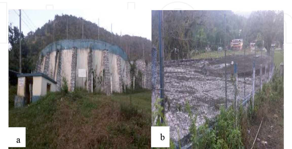
Figure 2. (a) An elevated rainwater concrete catchment of Elisabeth, Jamaica; (b) the surface runoff and the storage tank of Elisabeth, Jamaica RHI. (Adapted from Betasolo and Smith, 2017.)
