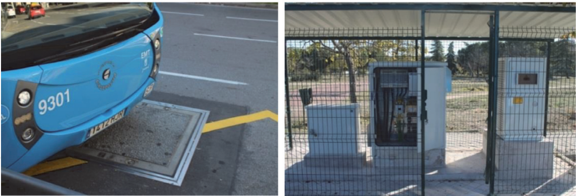
Figure 10. Bus charging by induction and necessary installations.
