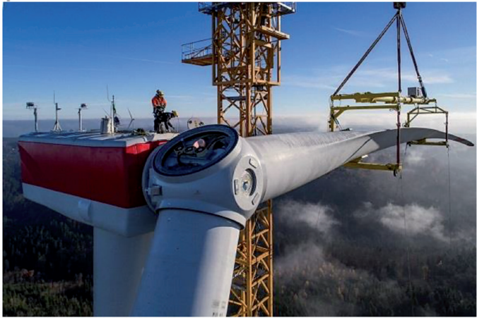
Figure 5. Installation of wind turbine blades on the tower in Gaildorf (Credit: Max Bögl (Holger Hessenthaler)).
