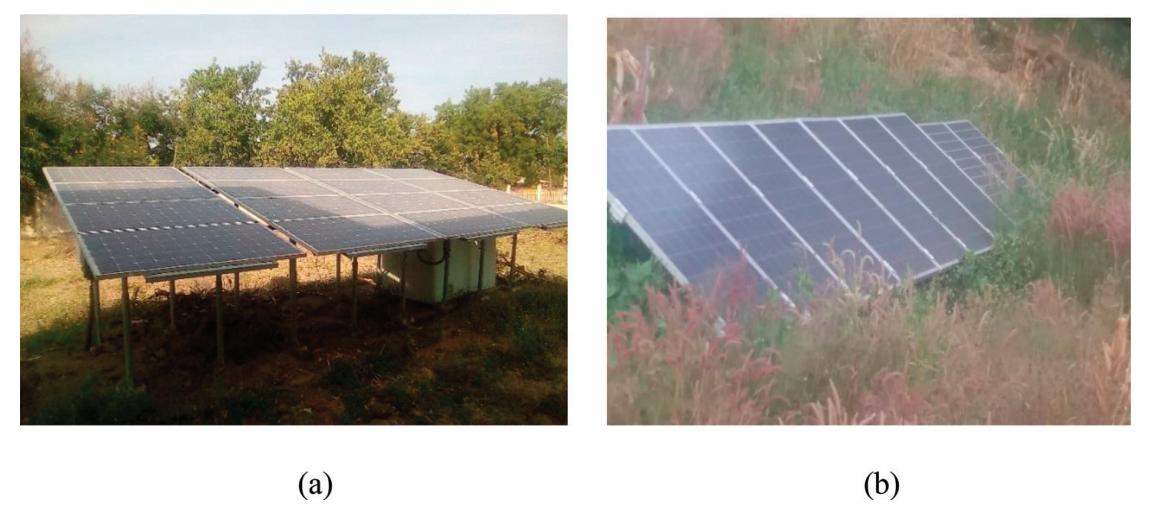
Figure 5. (a) Soiling and dust accumulation and (b) vegetation.
