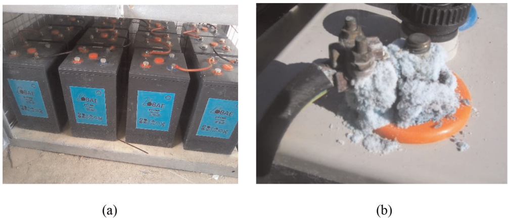
Figure 9. (a) Deep discharge of batteries and (b) sulfation of batteries due to lack of maintenance.
