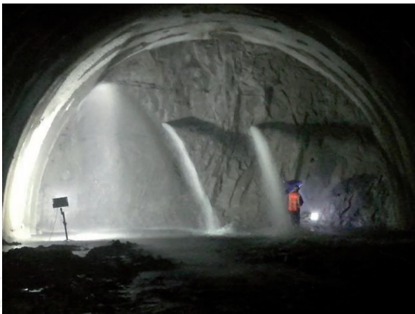
Figure 6. Water inrush in the tunnel after the advanced drilling.
