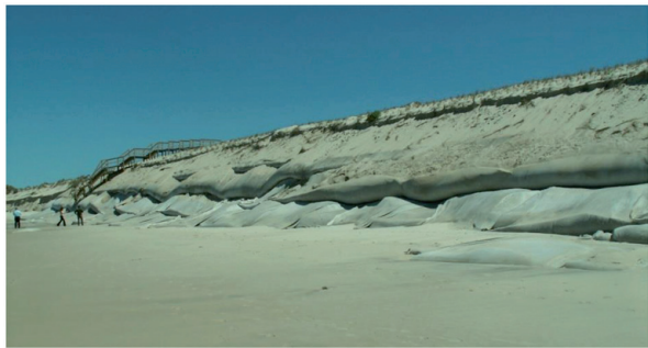
Figure 9. General aspect of some bottom geotextile layers after the high tides late in the winter of 2006, in April (Adapted from [12]).
