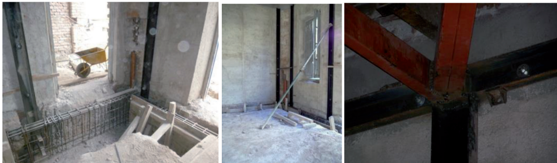
Figure 11. Reinforcement of foundations and reversible metallic structures in columns and lattice, Mitre school, 2012.
