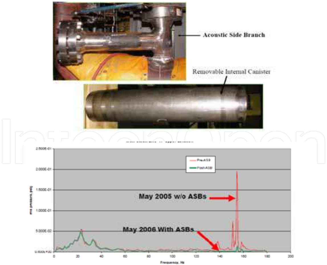
Fig. 16. Acoustic side branch, and the effect on the pressure, or load.
