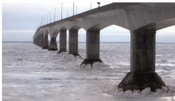
Figure 1. The ice cover around bridge piers (the confederation bridge, Prince Edward Island, 2015).
