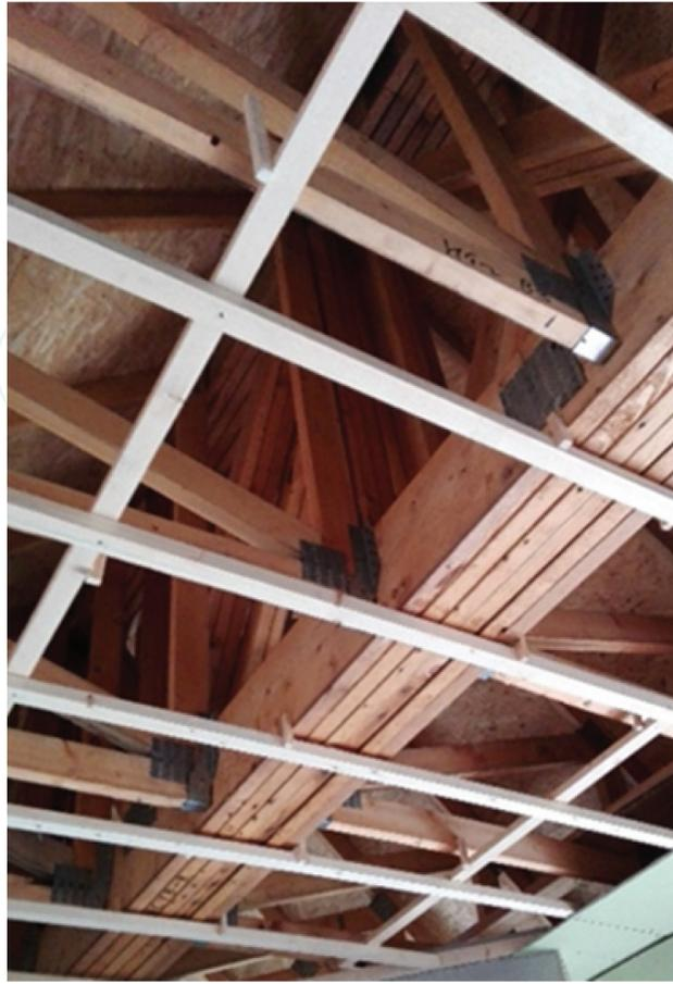
**Figure 1.** Application of girder truss in building structure.
