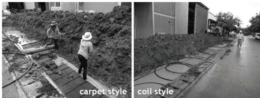
Figure 13. Installation of horizontal heat exchangers in Saraburi campus, Chulalongkorn University, Thailand (No. 7).
