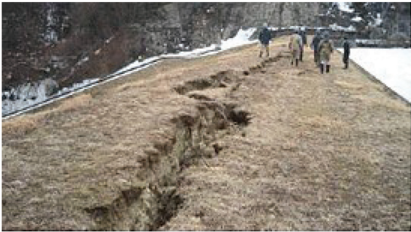
Figure 1. Crack at the Earth-fill dam.
