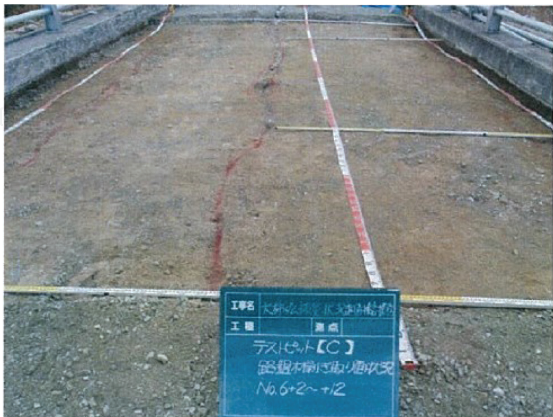
Figure 2. Crack at the rock-fill dam.
