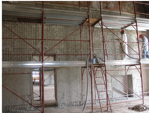
Figure 15. Application of mortar D as the reinforced plaster to Venaria's masonries.
