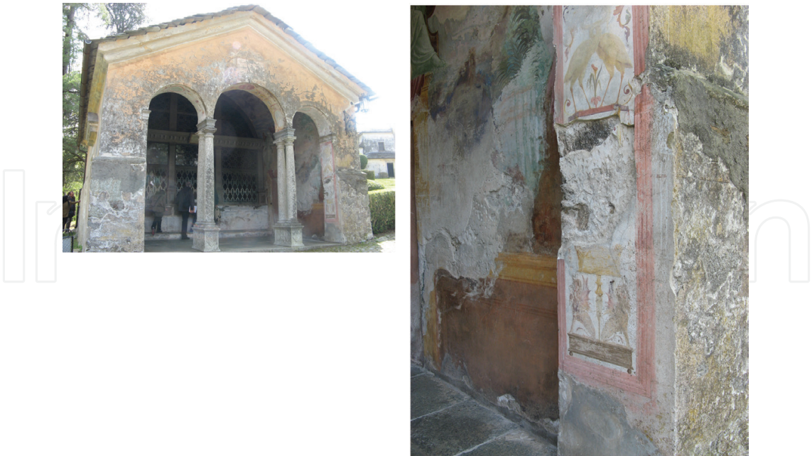
Figure 16. Decay of historical plasters because of the rain infiltrations (Sacro Monte of Varallo).
