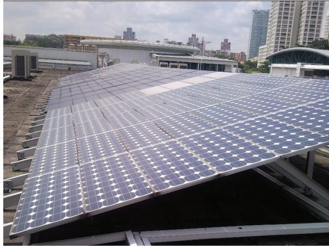
**Figure 7.** Conventional monocrystalline, polycrystalline and thin film (CIS) PV systems at CITI (BCA), Singapore [22].
