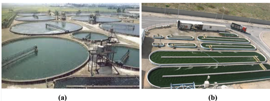
Figure 1. Open ponds cultivation system of microalgal cells. (a) Circular open pond and (b) raceway pond.
