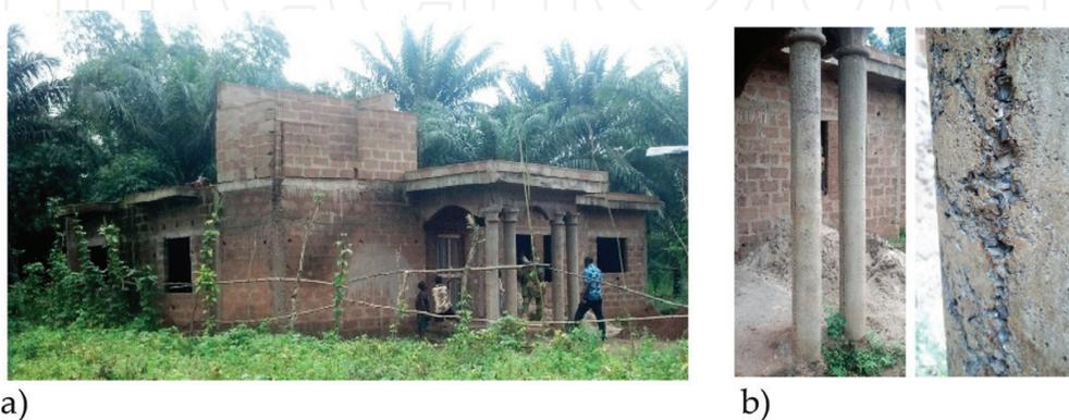
**Figure 1.** An example of a one-storeyed house in Misséréte, constructed in 2014 with the use of OPKS concrete for the supporting elements. (a) Overview of the ongoing building. (b) Zoom on the columns of the main facade, showing on their surface the oil palm kernel shells in the cement matrix.
