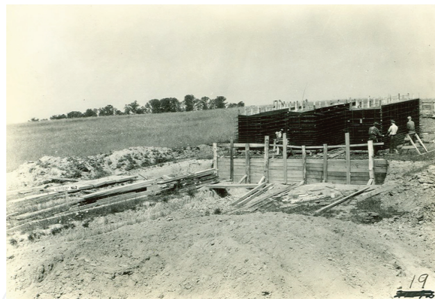
Figure 8. Construction and installation of three lysimeters at the NAEW.
