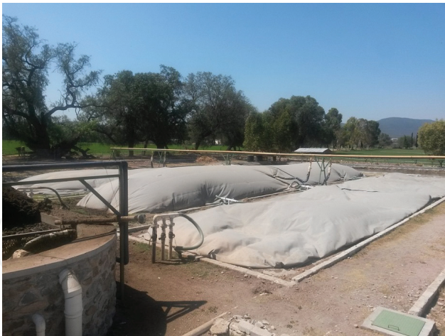
Figure 2. Covered lagoon digesters for cow manure treatment.
