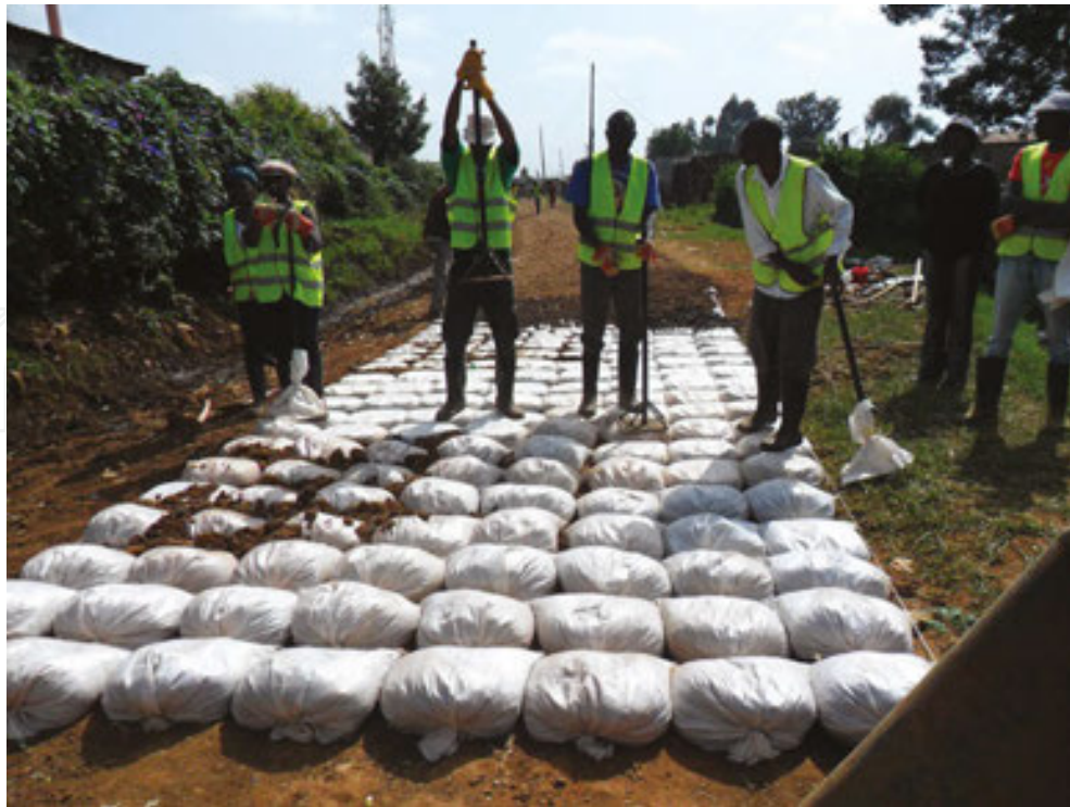
Figure 6. Practical manual compaction method for community work.
