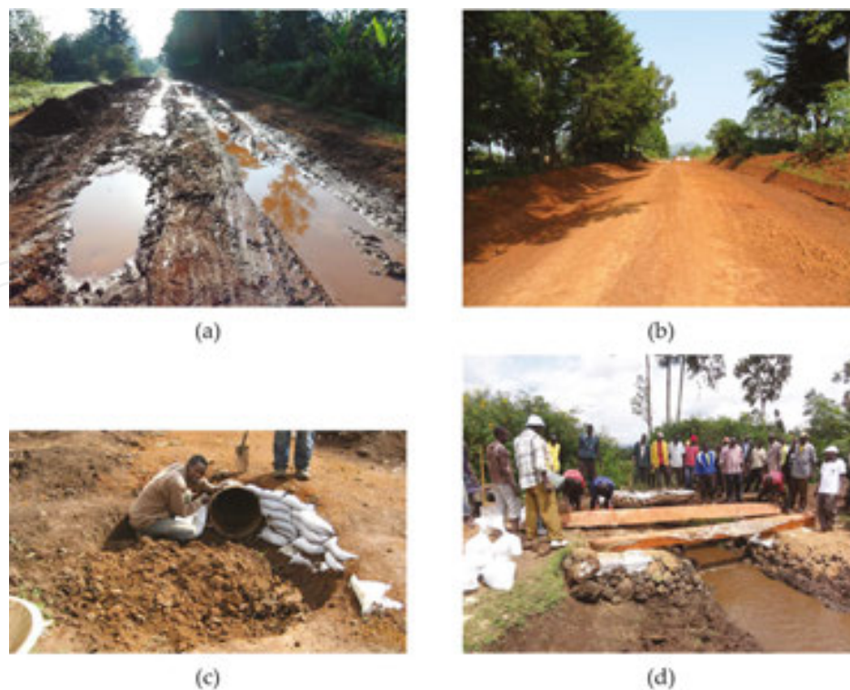
Figure 23. Applications of Do-nou technology during training/demonstrations with farmer groups: (a) Before construction; (b) after the construction; (c) retaining wall at inlet of culvert; (d) Do-nou abutment of wooden bridge.
