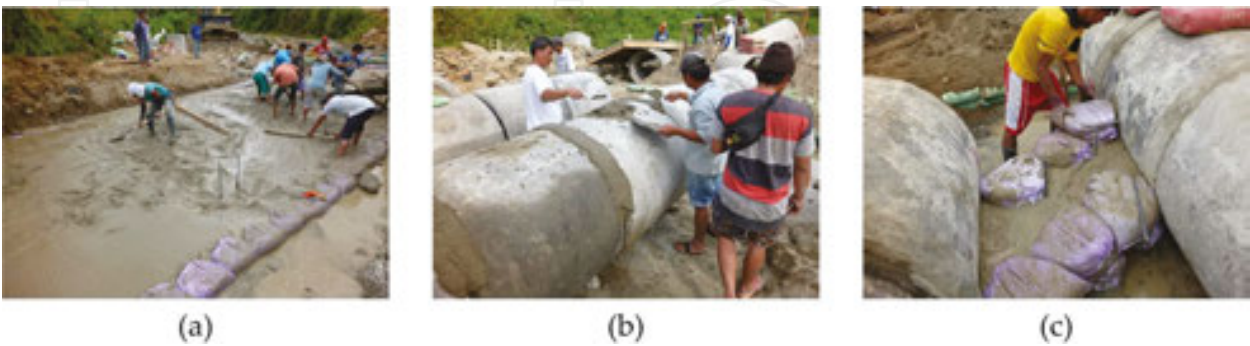
Figure 19. Work items managed by the community: (a) Leveling the concrete surface; (b) filling the gaps of RC pipes; (c) laying Do-nou.
