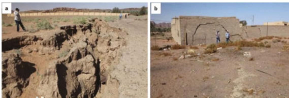
**Figure 3.** Photographic pictures showing (a) Earth fissures' distribution, (b) Impact of earth fissures on buildings.
