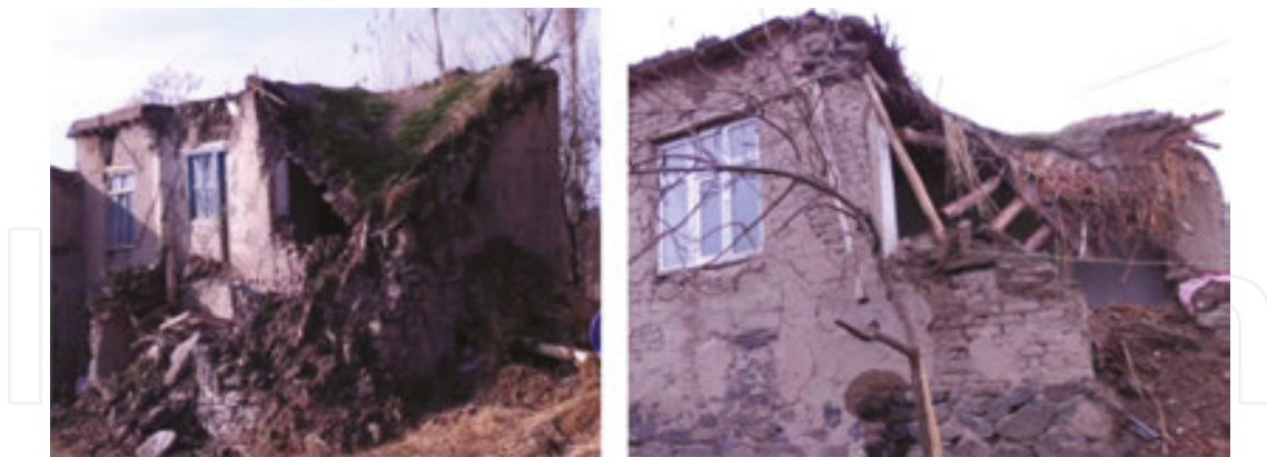
Figure 19. Damage to adobe structures due to heavy earthen roof during the Van earthquake [42].
