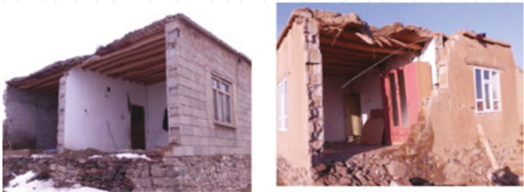
Figure 21. Out-of-plane mechanism of the briquette buildings [42].
