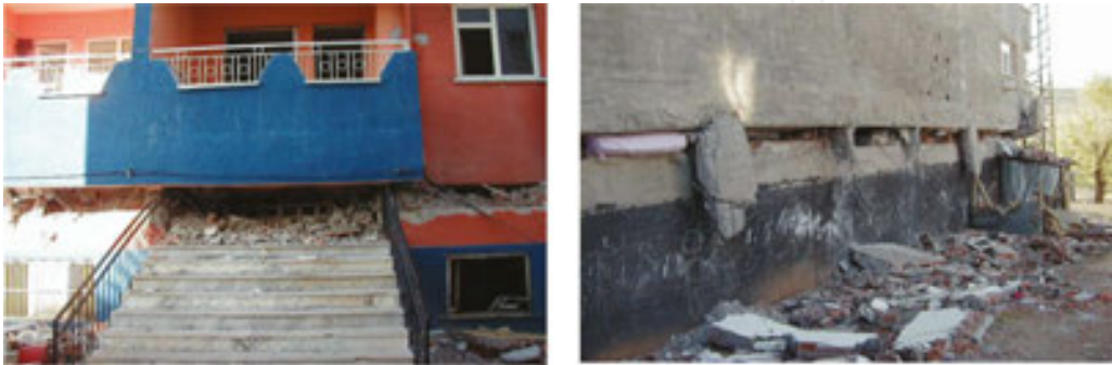
Figure 11. Weak storey mechanism during the Bingöl earthquake.
