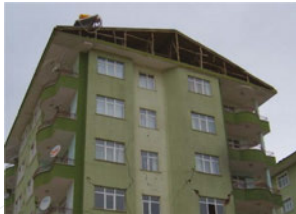
Figure 16. Failure of gable walls on top of the building during the Van earthquake.
