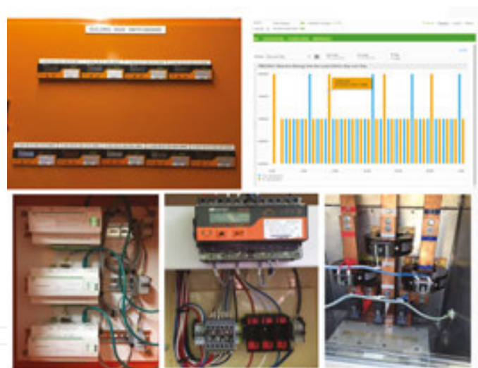
Figure 7. Installed Embedded Network Installations in 2015 at Murdoch University: from top left and left to right each row (a) 9× SATEC EM133 meters installed on main distribution board in one building, (b) chart showing output from the Schneider Electric COM510 energy server webpage, (c) showing the 3× energy servers with ethernet and modbus connections, (d) and (e) showing the EM133 smart meter installation using IPD CTs, test links and voltage fuses.
