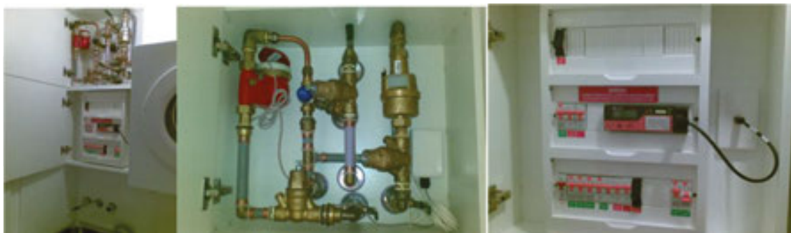
Figure 9. Meters installed at Central Park: (a) typical complete installation of meters for gas, electricity, hot water, cold water, (b) close up view of the gas and water meters, (c) showing electricity meter EM133AR installed in residential DB with Ethernet output to building IP backbone.
