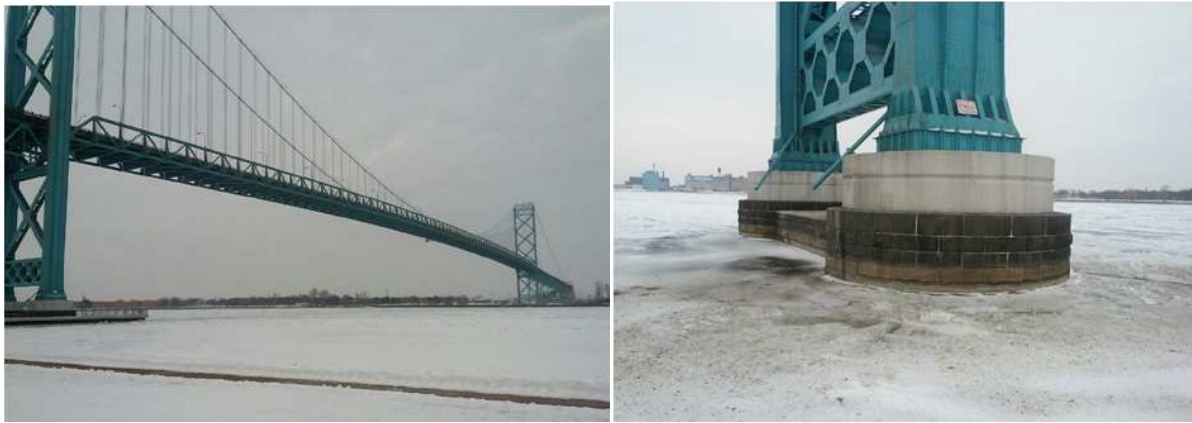
Figure 1. The ice cover around bridge piers (Ambassador Bridge, Windsor, ON, Canada, 2015)
